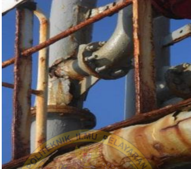
Gambar 1.11 Vacuum Valve bocor
