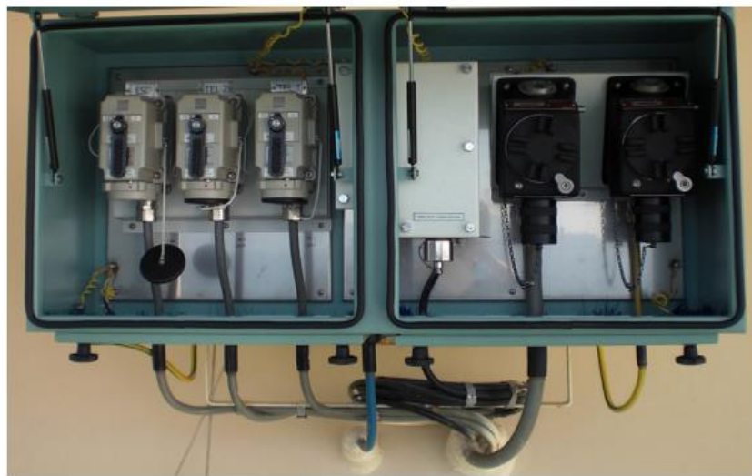
Gambar 2.9. Optical Cable Box
