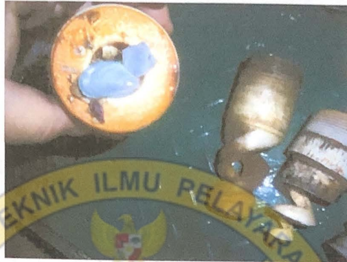
Gambar kondisi nozzle cooling spray sea water tersumbat
