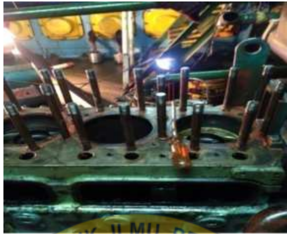
Gambar . Top overhaul diesel generator
