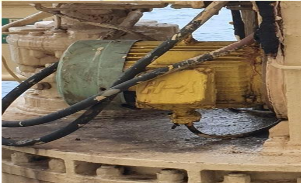
Motor listrik provision crane
