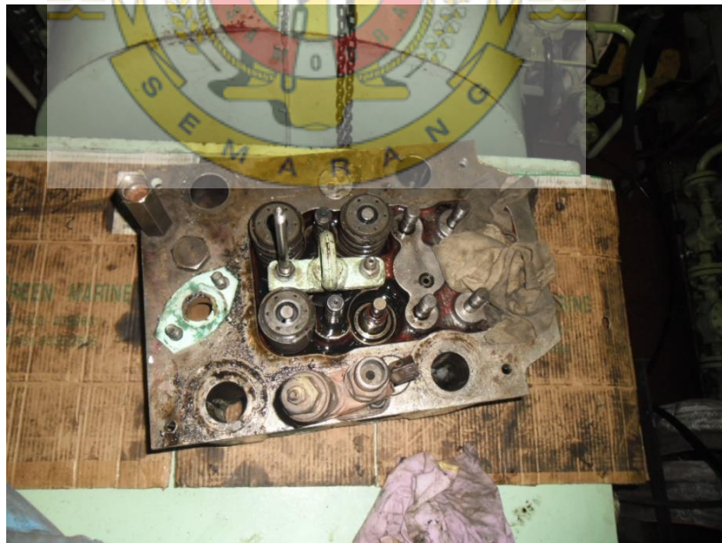
Gambar 4 Proses Overhaul Cylinder head generator
