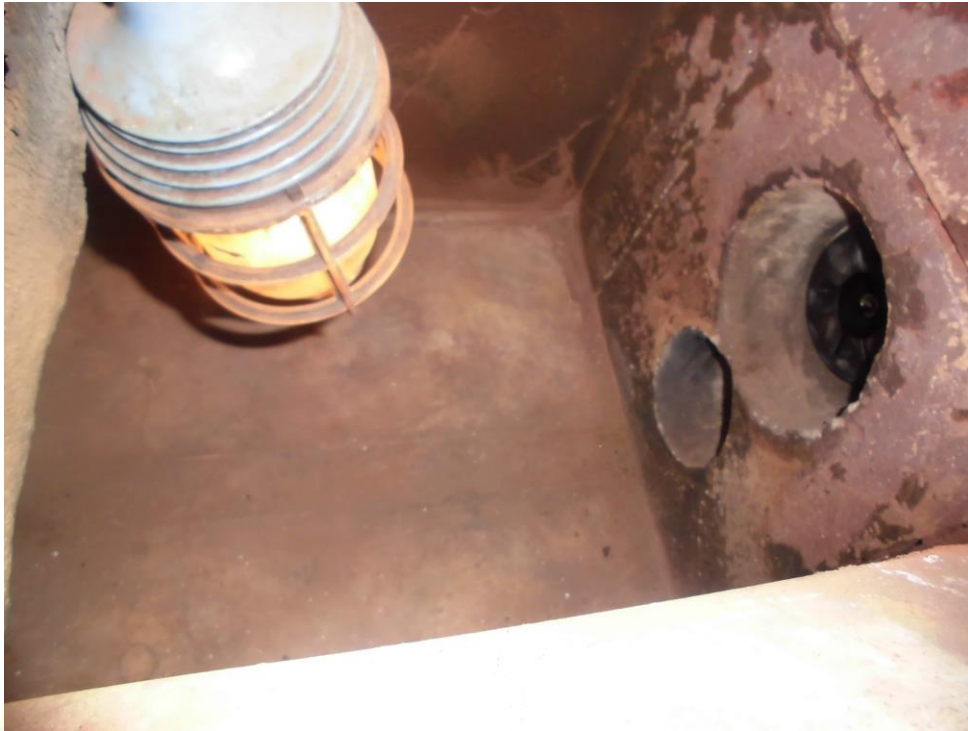
Gambar cleaned furnace of incinerator
