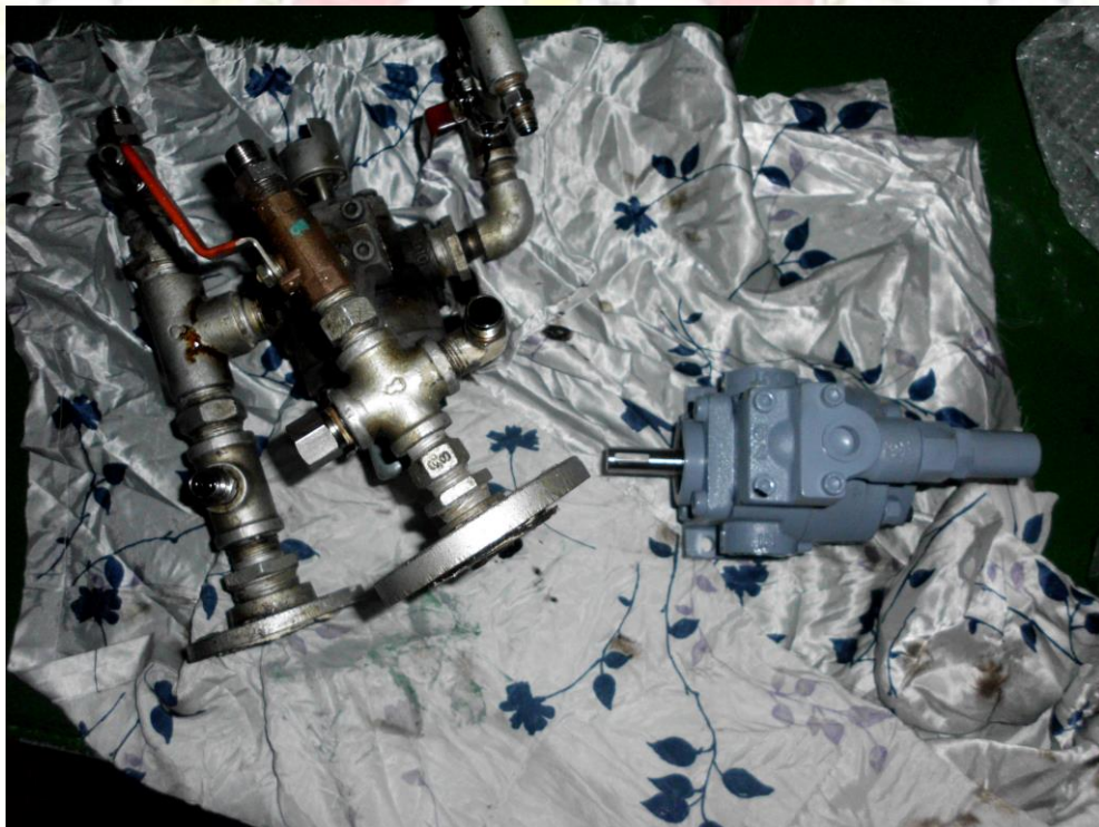
Gambar overhaul trochoid pump of incinerator
