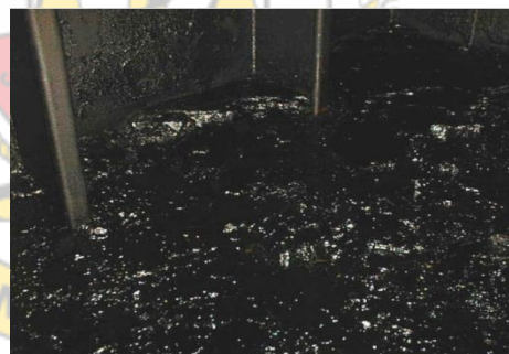
Gambar 2.8. Fuel Oil Incompatibility terjadi pada storage tank Sumber: dokumentasi fuel handling and storage problem on MV. Cap Bon (2011)
