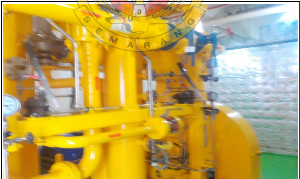
Cargo compressor LPG/C Gas Arar
