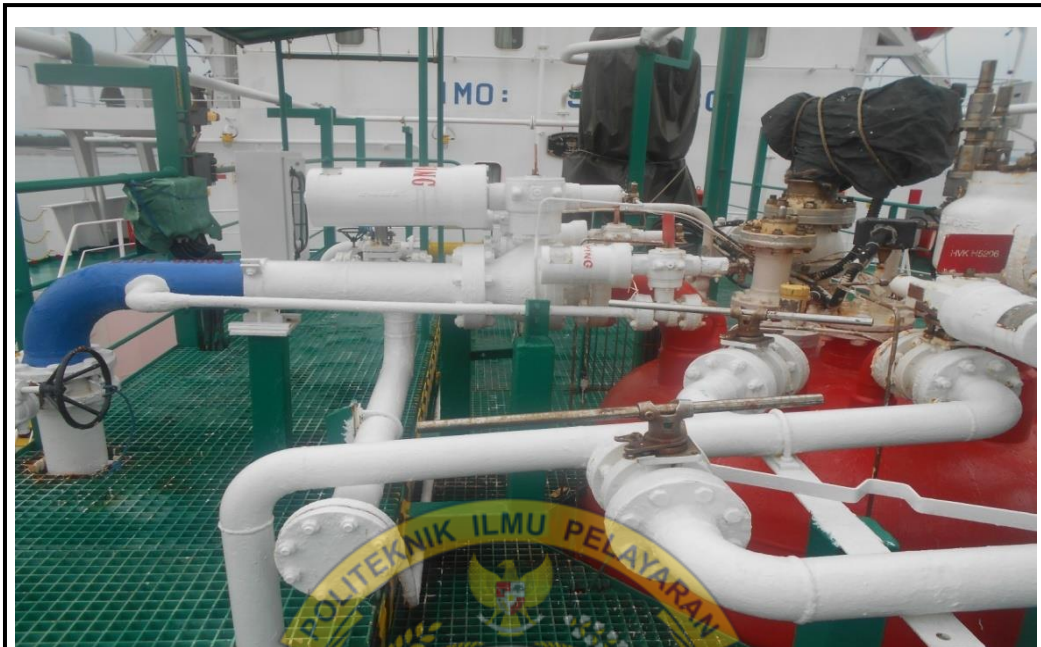
Pipe line discharge dan safety relief valve
