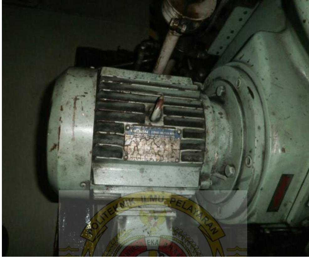
Gambar. 3 electric motor fuel oil purifier
