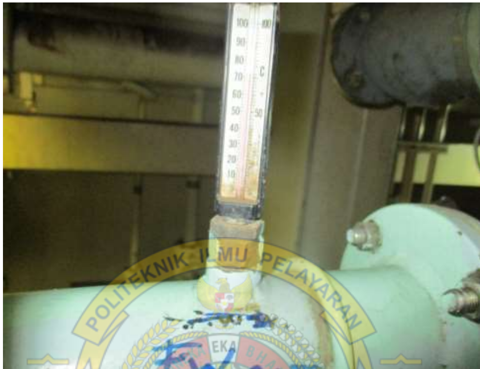
Gambar 13 Thermometer fresh water out main engine
