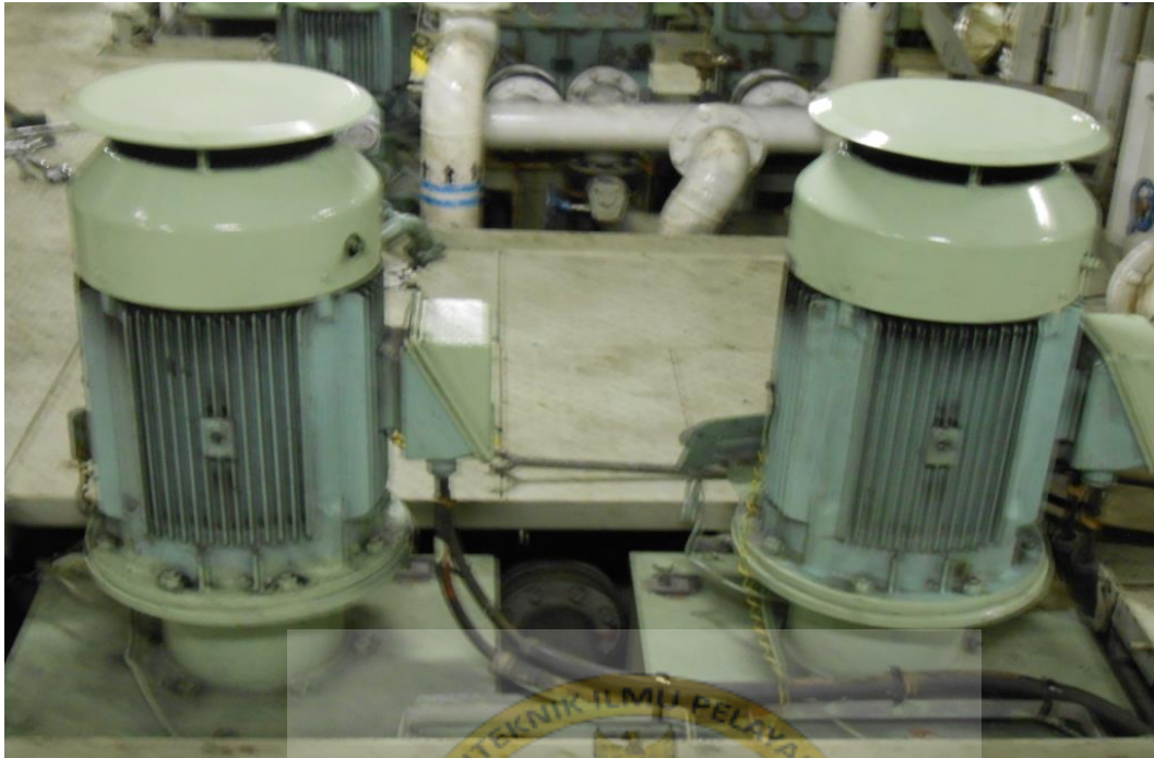
MAIN SEA WATER COOLING PUMP
