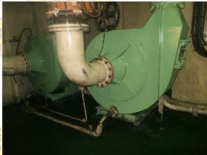
Gambar 2.4. Blower Inert Gas System
