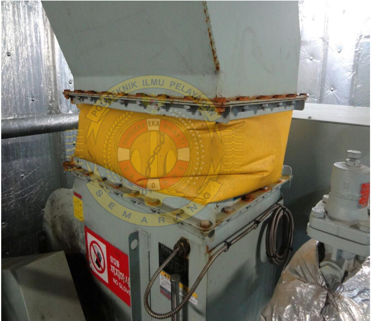
Gambar flexible connection Air Handling Unit
