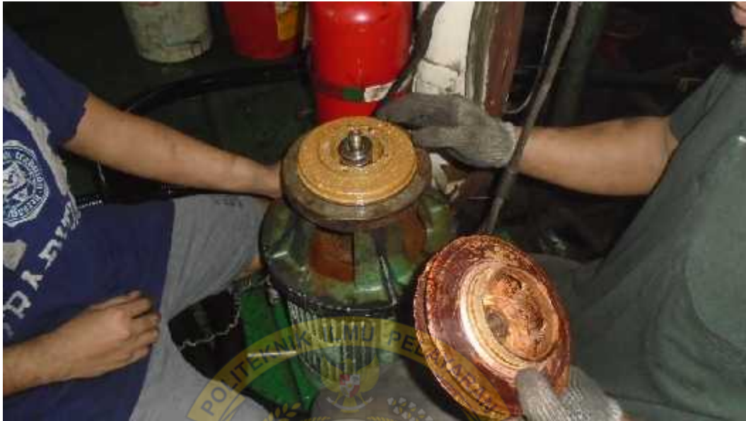
Gambar : Overhaul boiler feed water pump di MV. Sinar Praya
