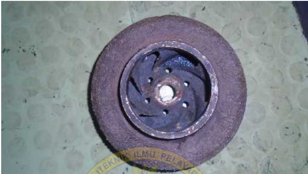
Gambar : Kavitasi pada impeller boiler feed water pump di MV. Sinar Praya
